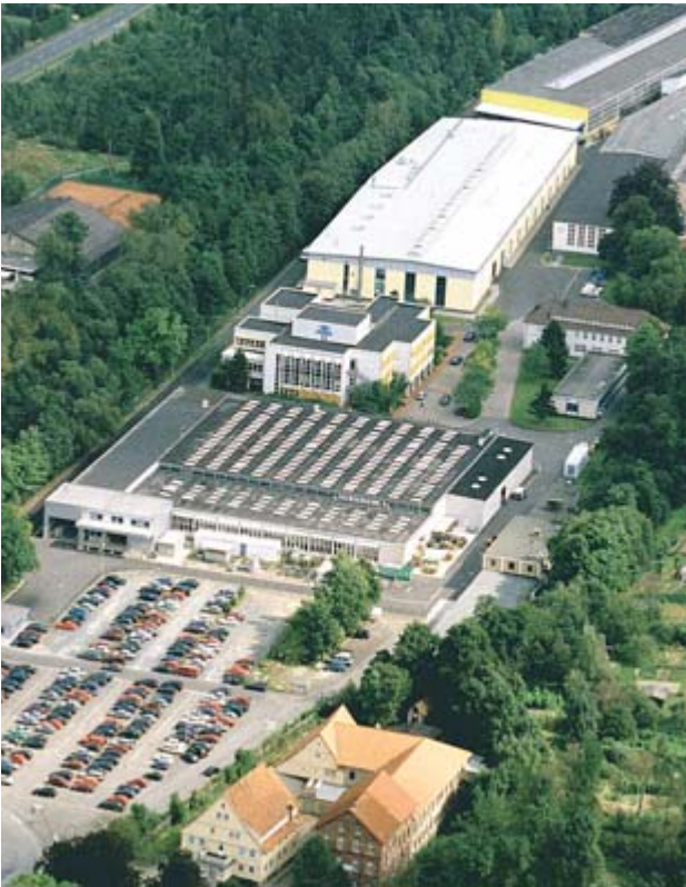
Piller Headquarters & Manufacturing Facility, Osterode
