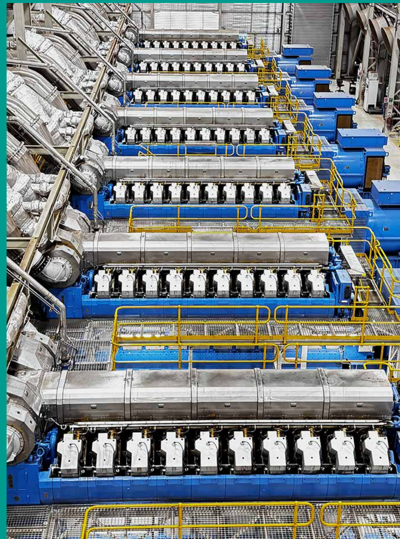
ABOVE: ON LAND. 15 Bergen gas engines power Ironbridge magnetite mine in Western Australia, integrating 170MW of medium speed genset power with 150mw solar power.
