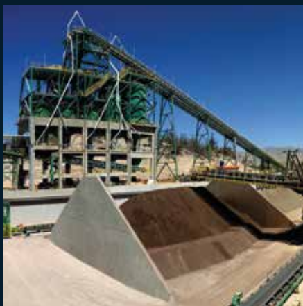
Claudius Peters Limestone Bridge Reclaimer, North Africa
