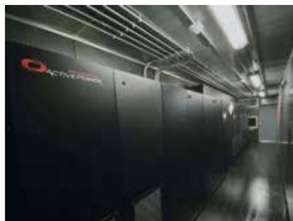
Active Power Inc.'s Powerhouse™ – up to 1.2MW of 'plug & play' UPS built into a standard 40-foot (12 metre) ISO container.
